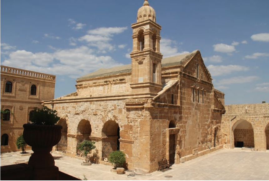
Fig. 3.3.11 Monastery of Mor Yaʿqub at Şālah, main church
